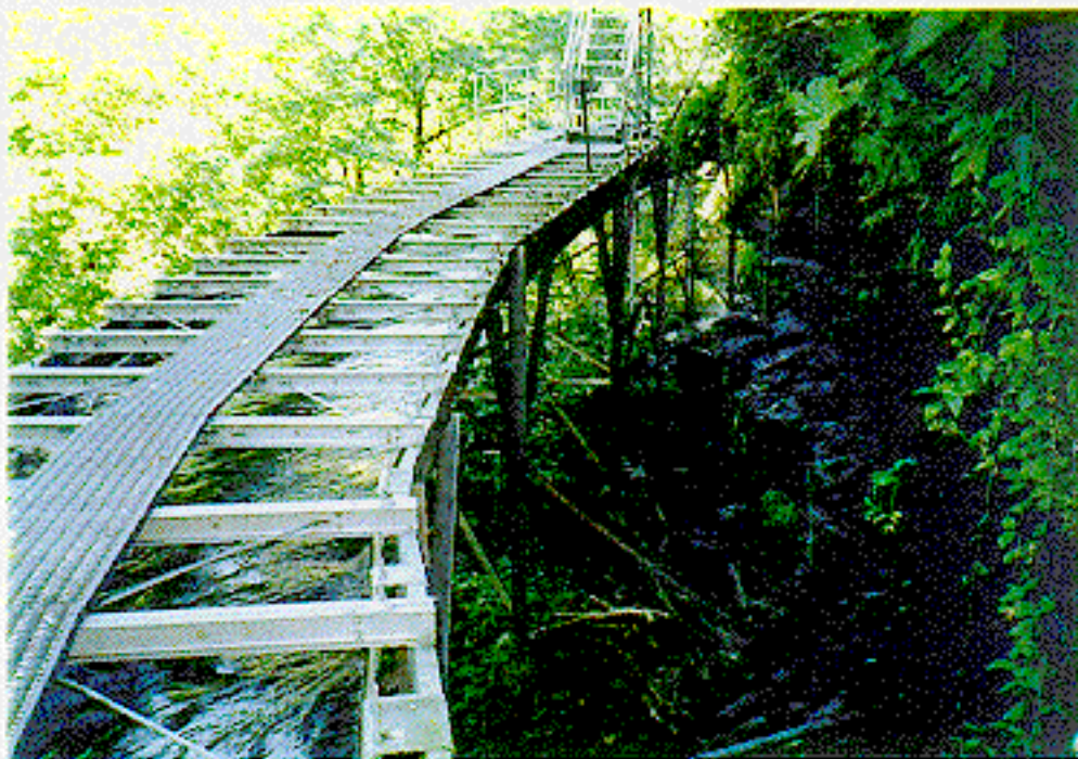
Photograph 6. - Eagle Canyon Canal: Metal flume section and stairway.
