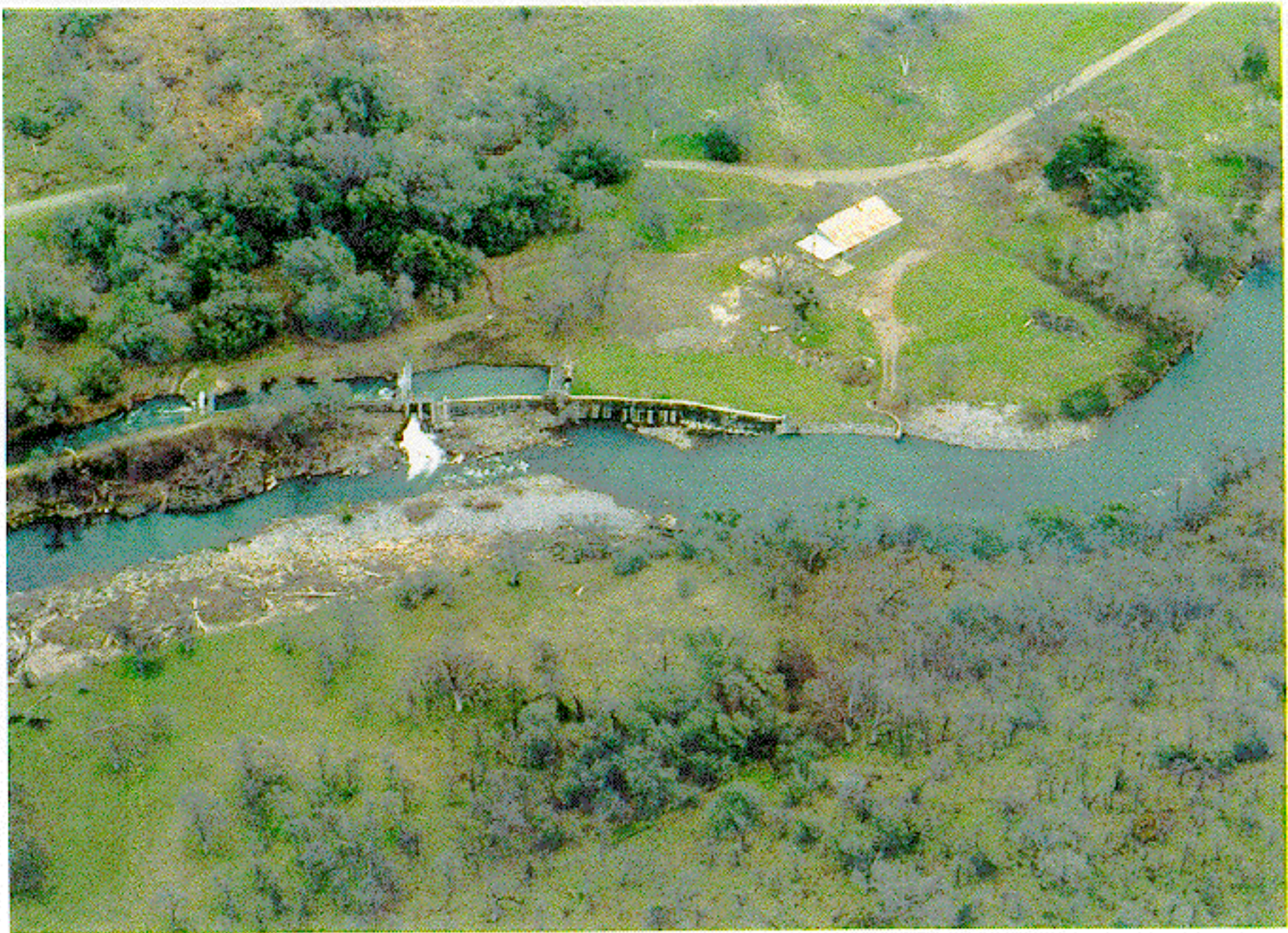
Photograph E-6. Coleman damsite after dam removal.
