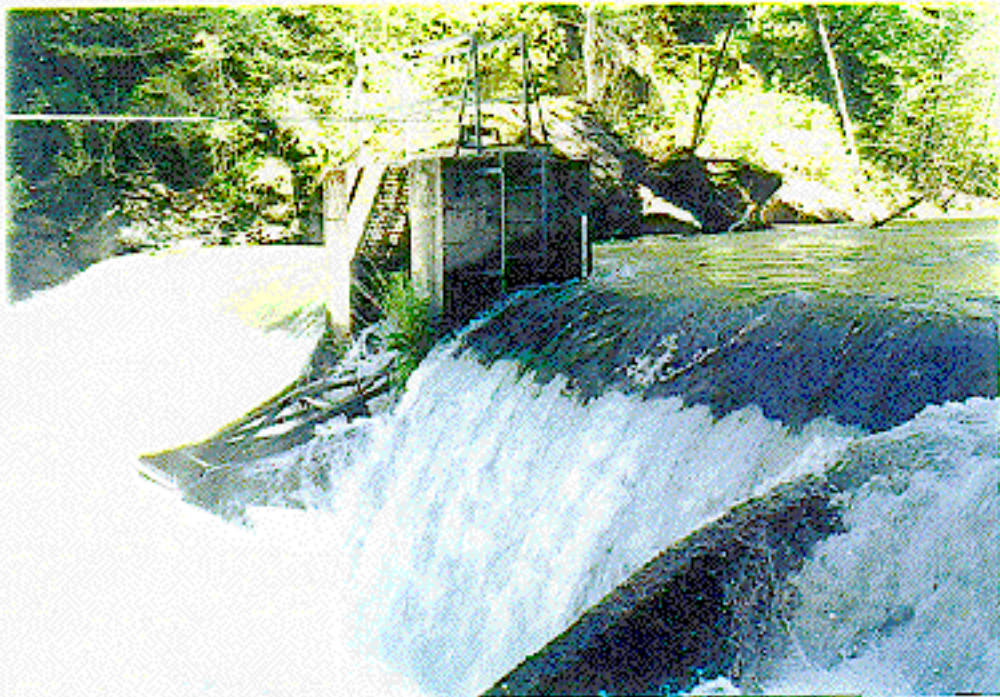
Photograph 2. - Eagle Canyon Dam: 4-by 10-foot radial gate sluiceway
