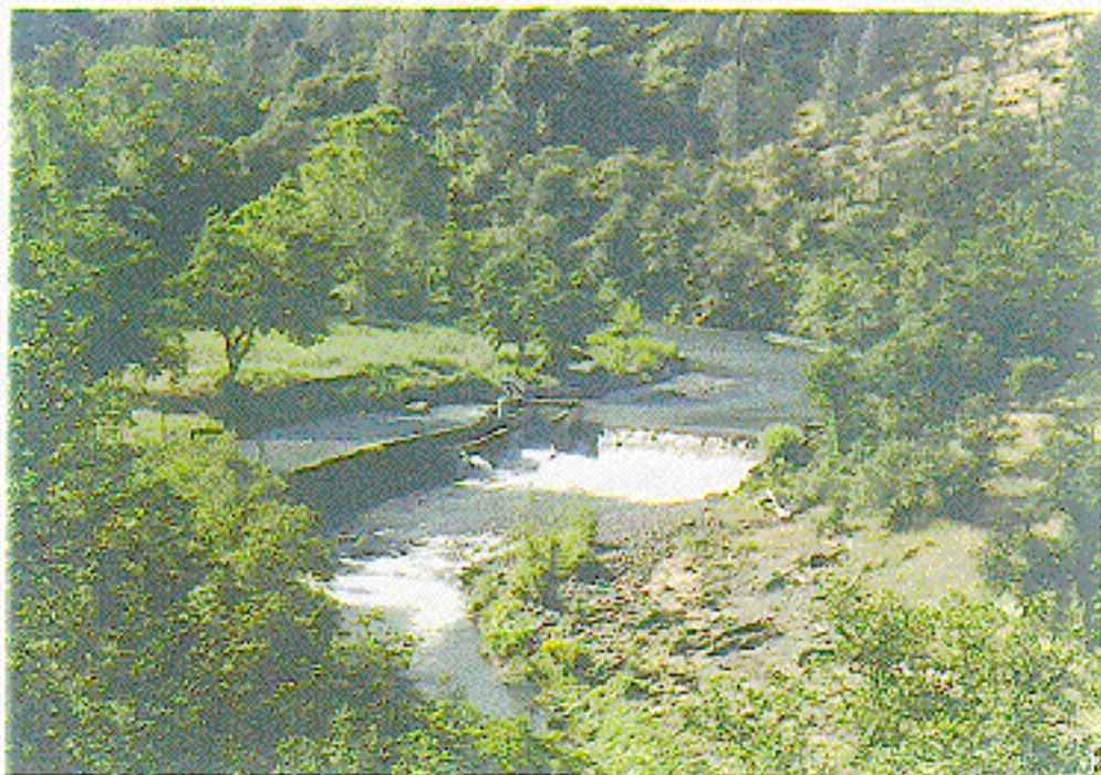
Photograph 15 - Coleman Dam. Existing dam and associated facilities.
