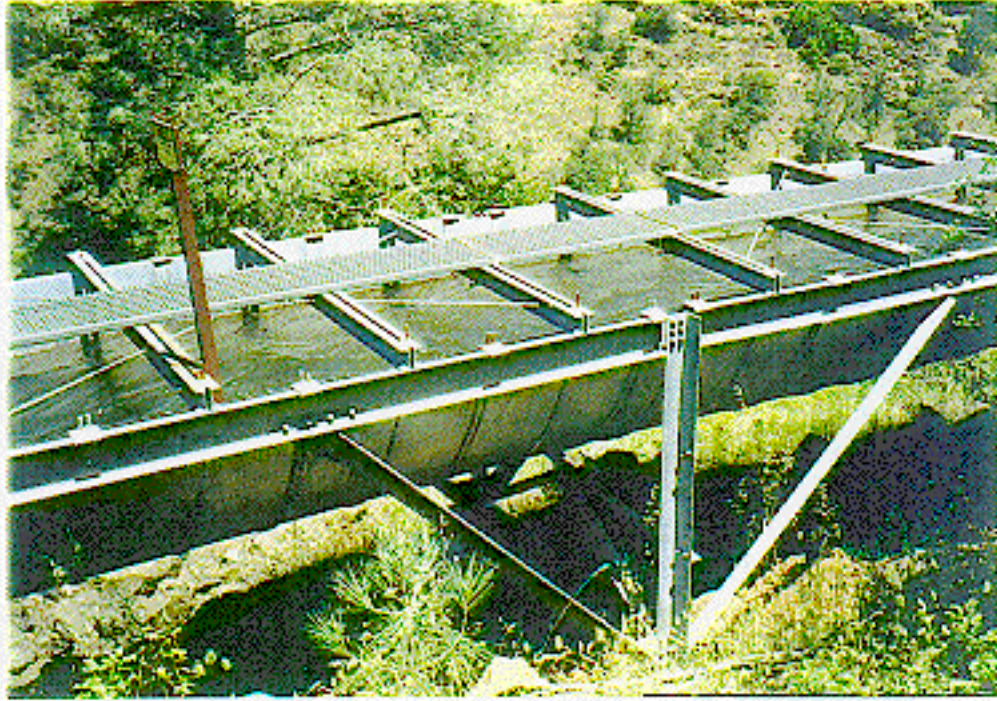
Photograph 7. - Eagle Canyon Canal. Metal flume section side view.
