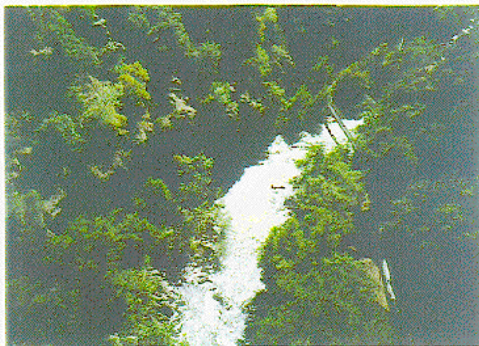
Photograph 13. - Wildcat Canal: Pipeline crossing North Fork.
