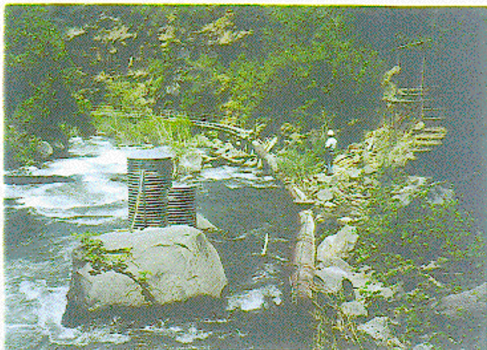
Photograph 11. - Wildcat Canal: Pipeline and handrails
