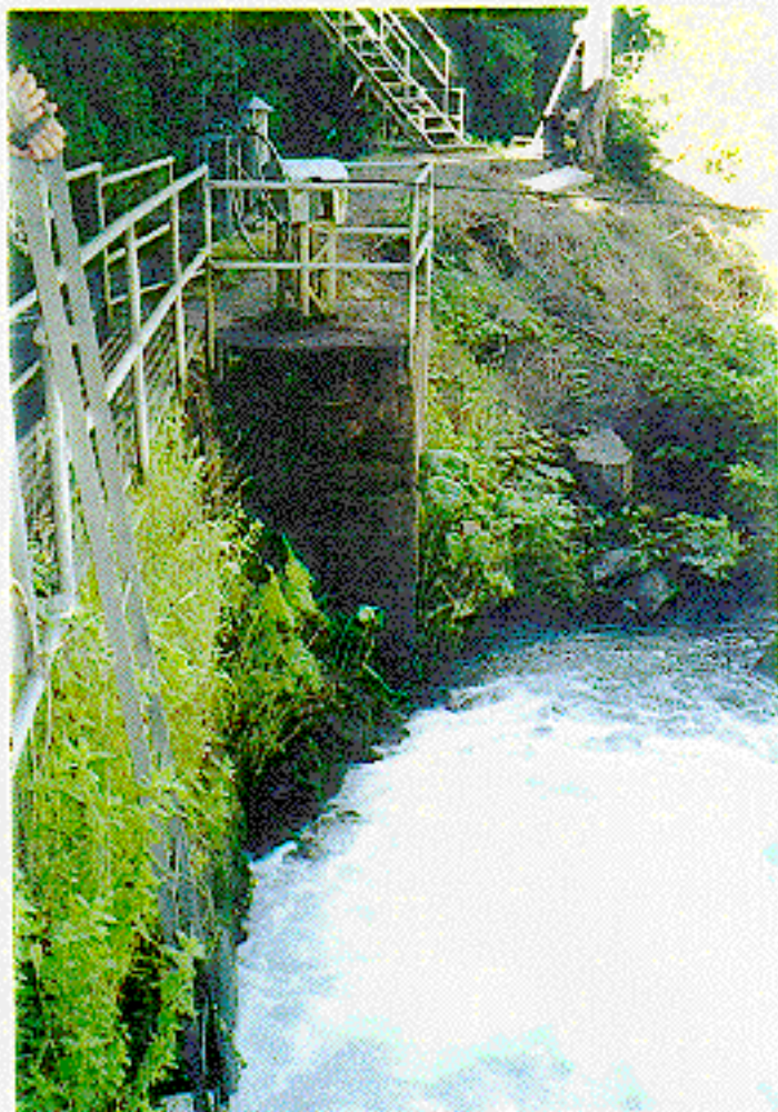
Photograph 4. - Eagle Canyon Dam. Canal wall and gate winch block.
