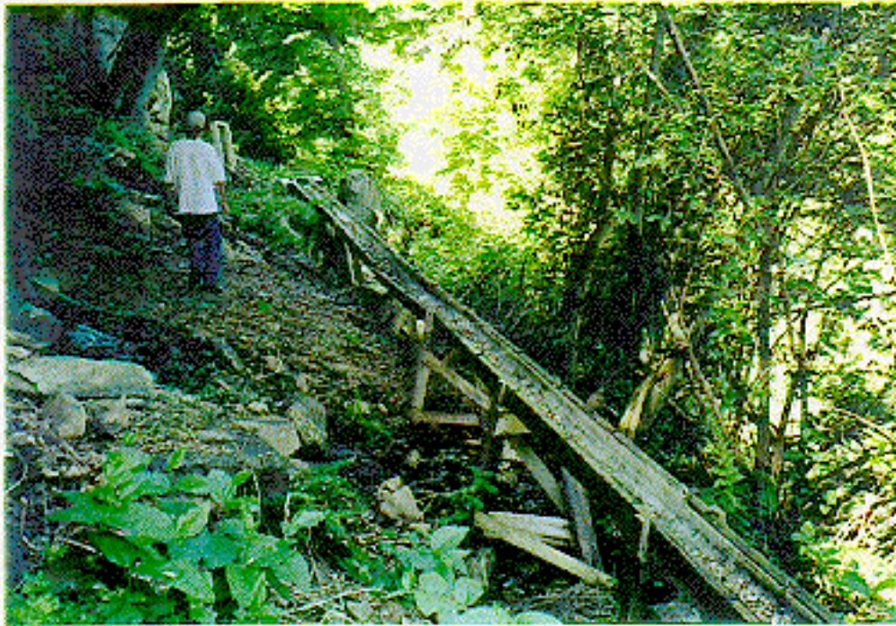
Photograph 8. - Eagle Canyon Dam. Small flume section for spring flows
