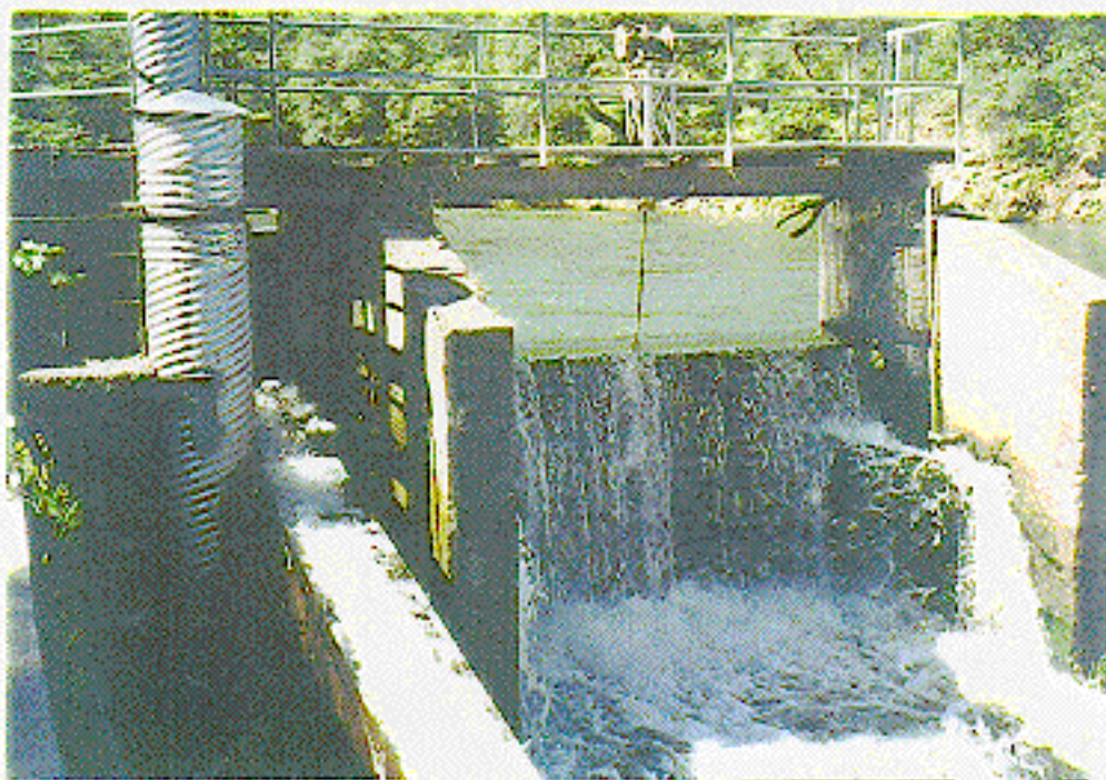
Photograph 18. - Coleman Dam: 14-by 8-foot radial gate sluiceway and fish ladder
