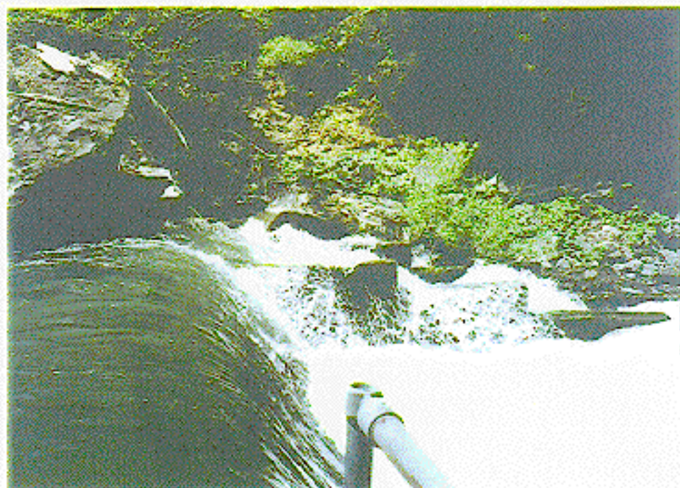
Photograph 12. - Wildcat Dam: Nonoverflow section and fish ladder structure
