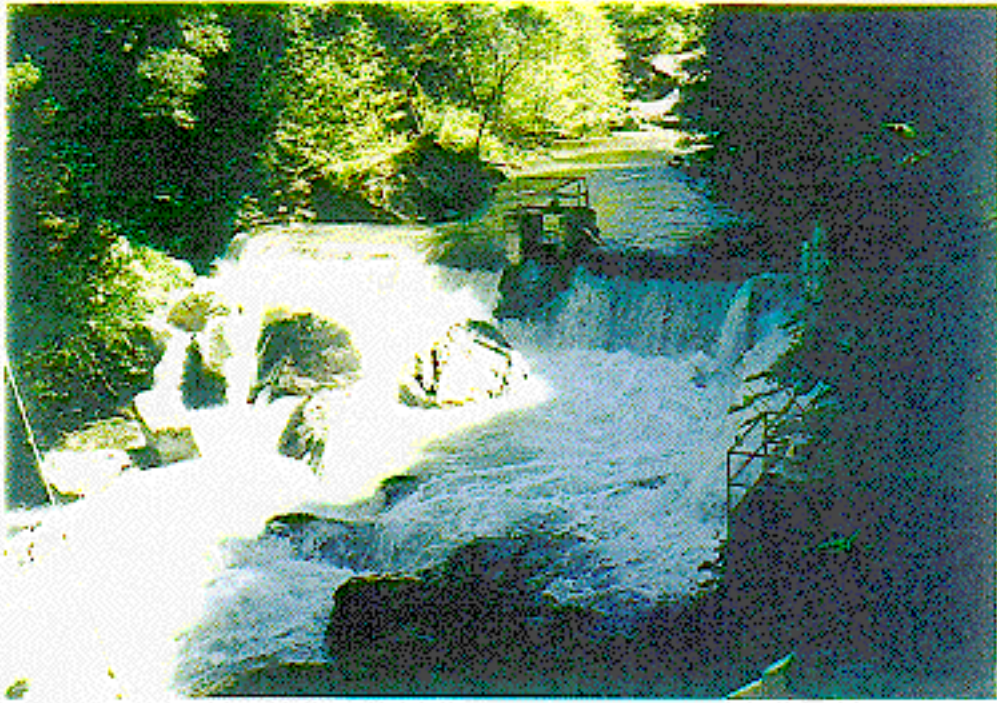
Photograph 1. - Eagle Canyon Dam: Existing dam and associated facilities.
