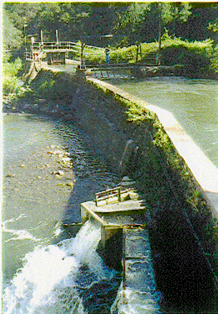
Photograph 20. - Coleman Canal Masonry wall, looking downstream.
