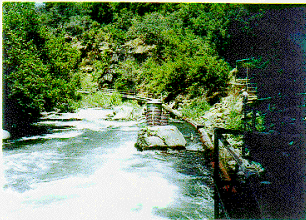
Photograph 10. - Wildcat Dam: Right abutment canal intake and access footbridge in foreground.
