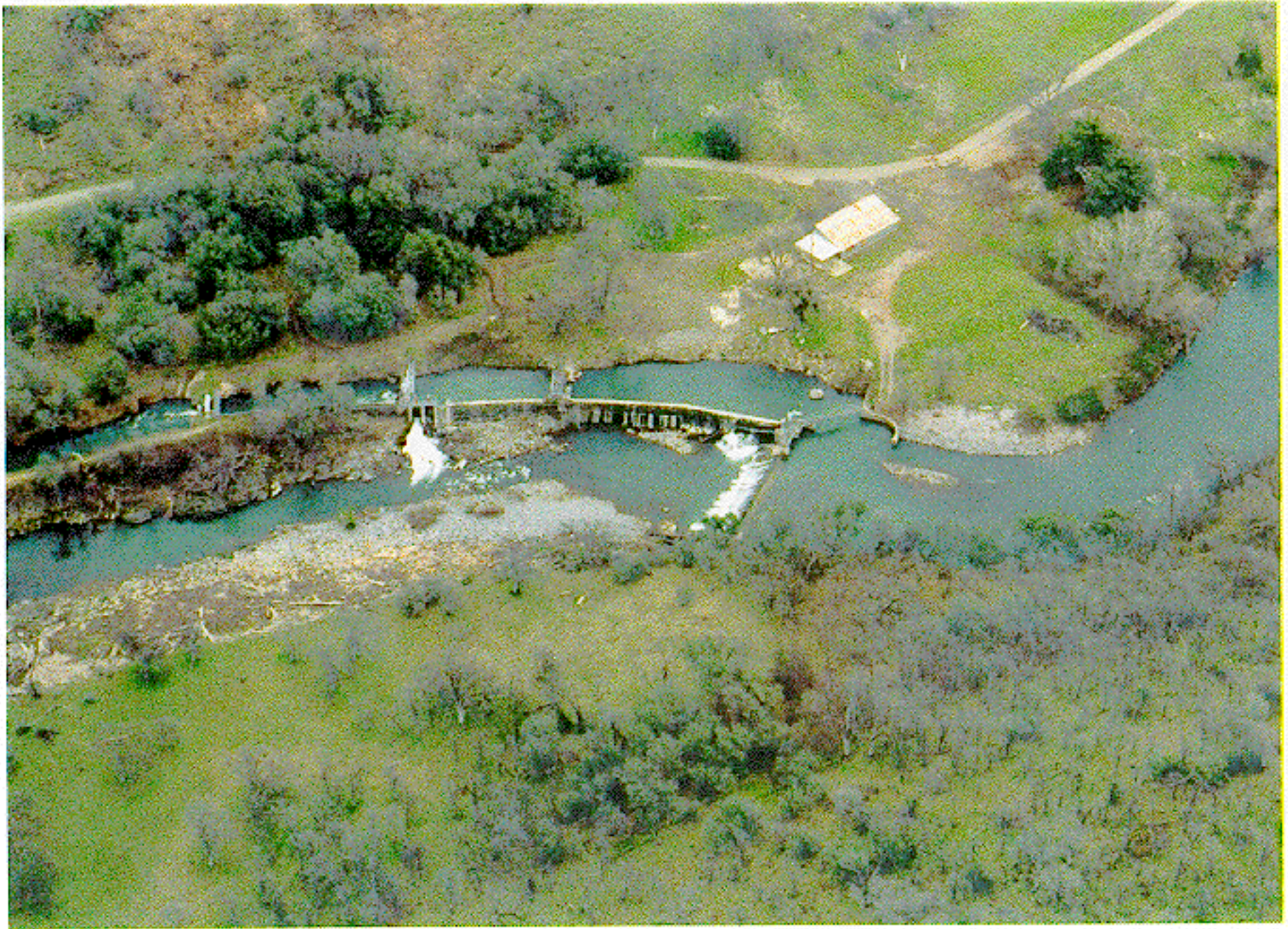
Photograph E-5. Coleman Dam (existing conditions).
