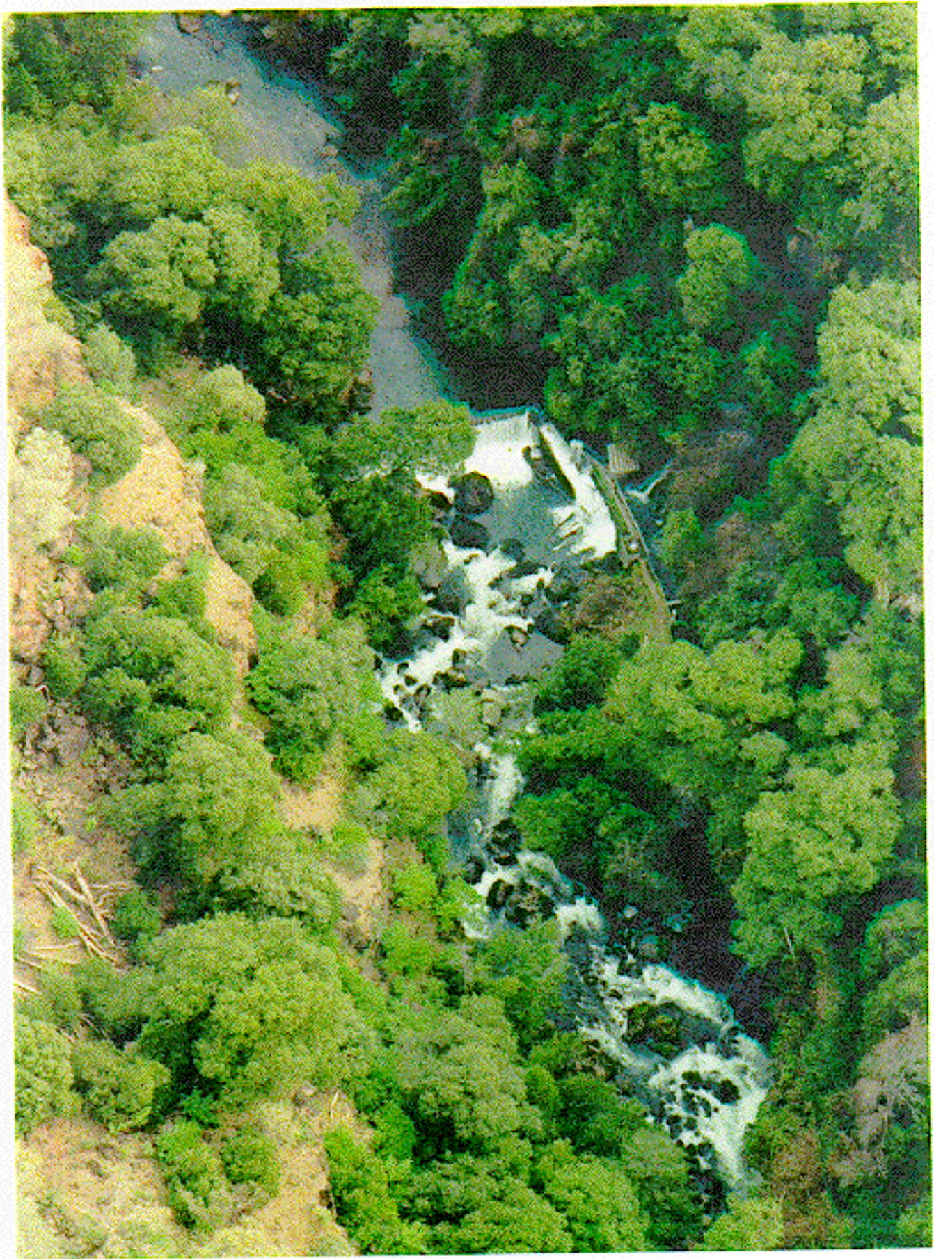
Photograph E-3. Eagle Canyon Dam (existing conditions).
