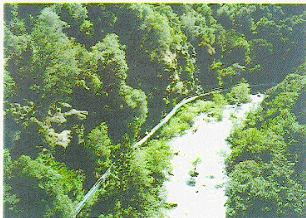
Photograph 14. - Wildcat Canal: Pipeline with handrails, along North Fork.
