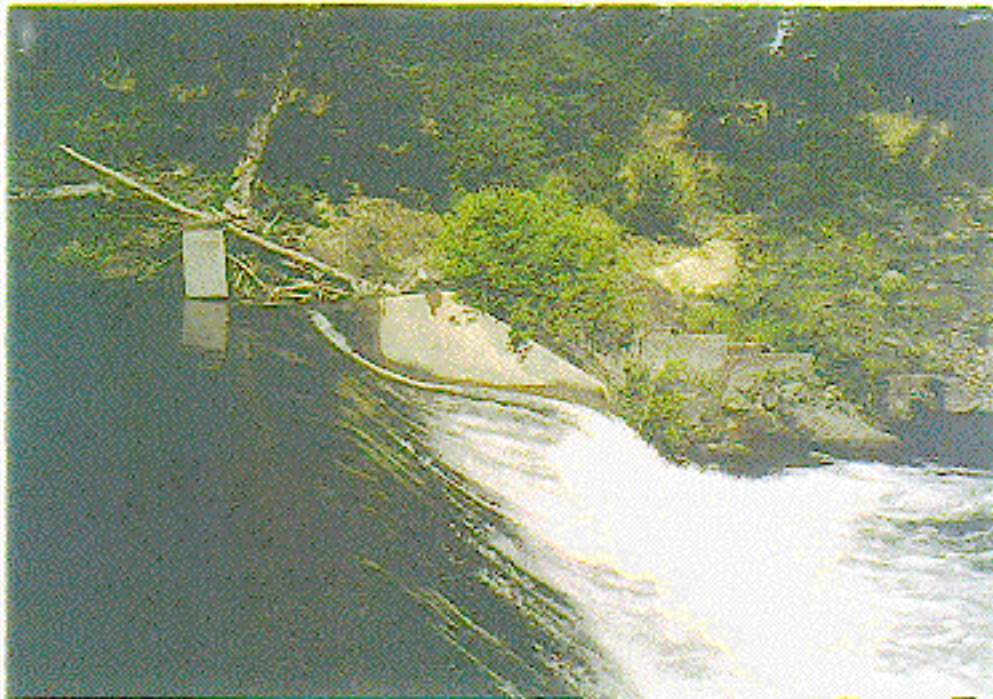
Photograph 17. - Coleman Dam. Left abutment head wall, training wall, and original fish ladder.
