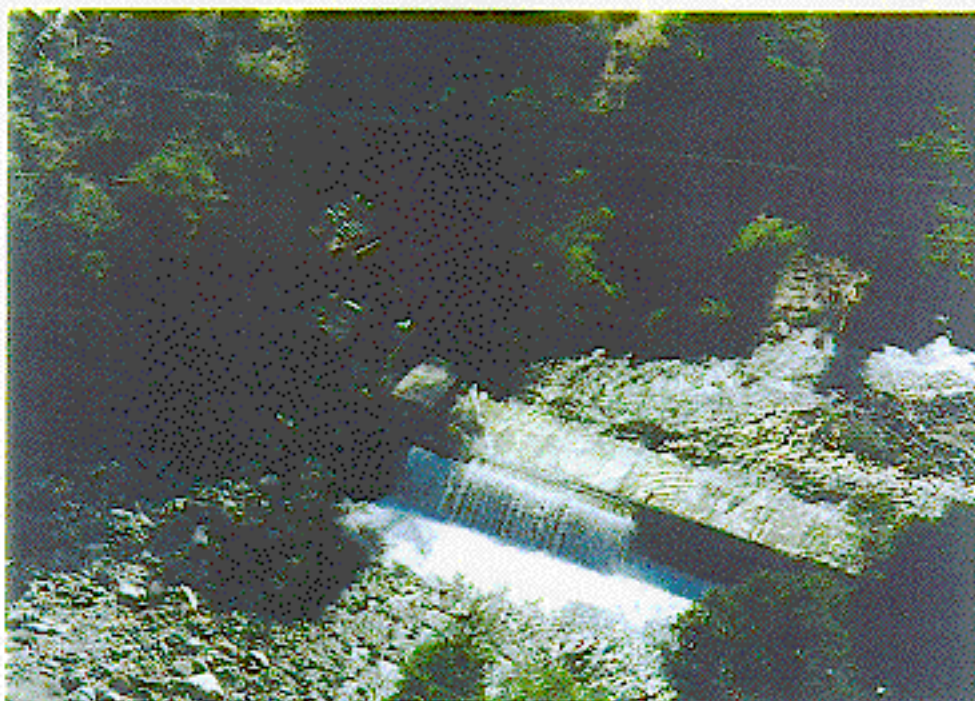
Photograph 4. - South Diversion Dam: Overflow crest and right abutment features.
