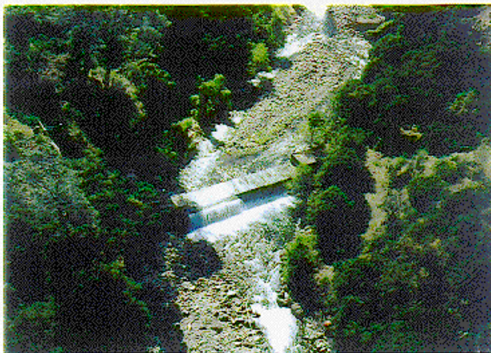
Photograph 1. - South Diversion Dam: Aerial view of existing dam, looking upstream.
