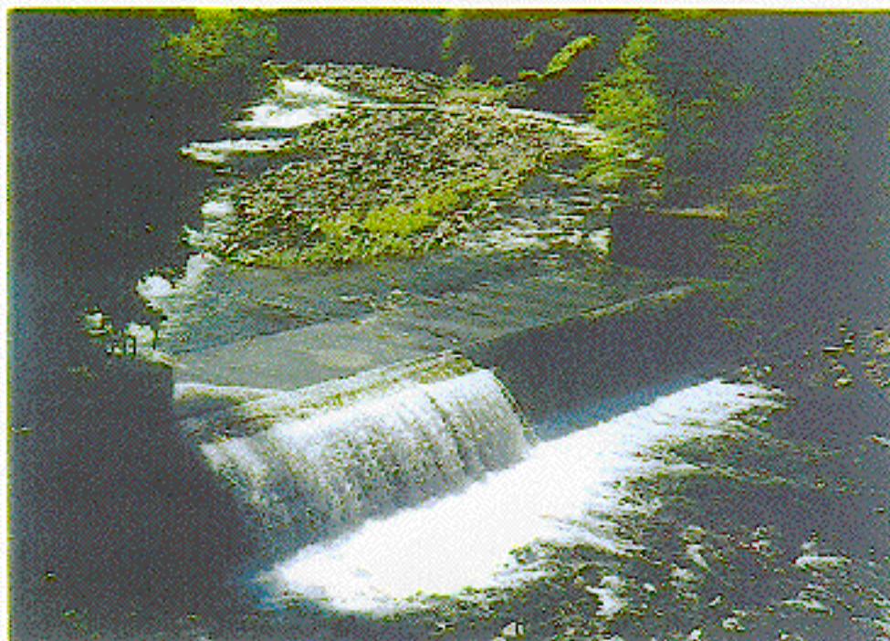
Photograph 3. - South Diversion Dam: Overflow crest and left abutment nonoverflow section.
