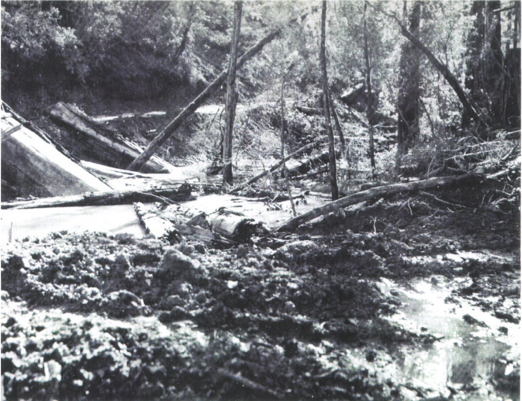
NORTH FORK, GARCIA RIVER, MENDOCINO COUNTY, intersection of a small tributary, Nov. 22, 1955. Landing and parking area built into confluence. Mud in foreground is shoulder of parking area, looking upstream into tributary. No culvert apparent and water appears to be seeping under logs and rubble. No flow visible into the Garcia. ( Fish and Game photo. )
