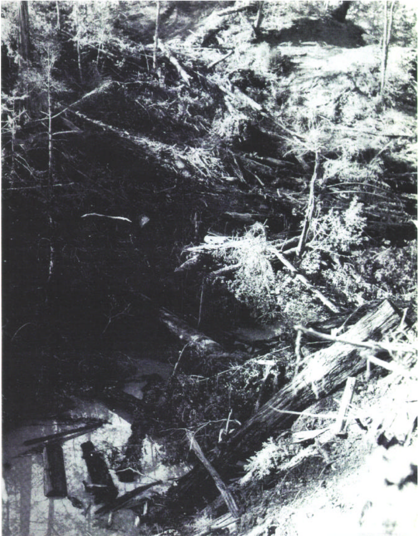
NORTH FORK, GARCIA RIVER, MENDOCINO COUNTY, Nov. 22, 1955. Stream bed blocked. Side hill left with skid roads running into stream bed without water checks; covered with debris which will be washed into stream by heavy runoff. Rubble which blocked stream was pushed off road by operator. ( Fish and Game photo. )
