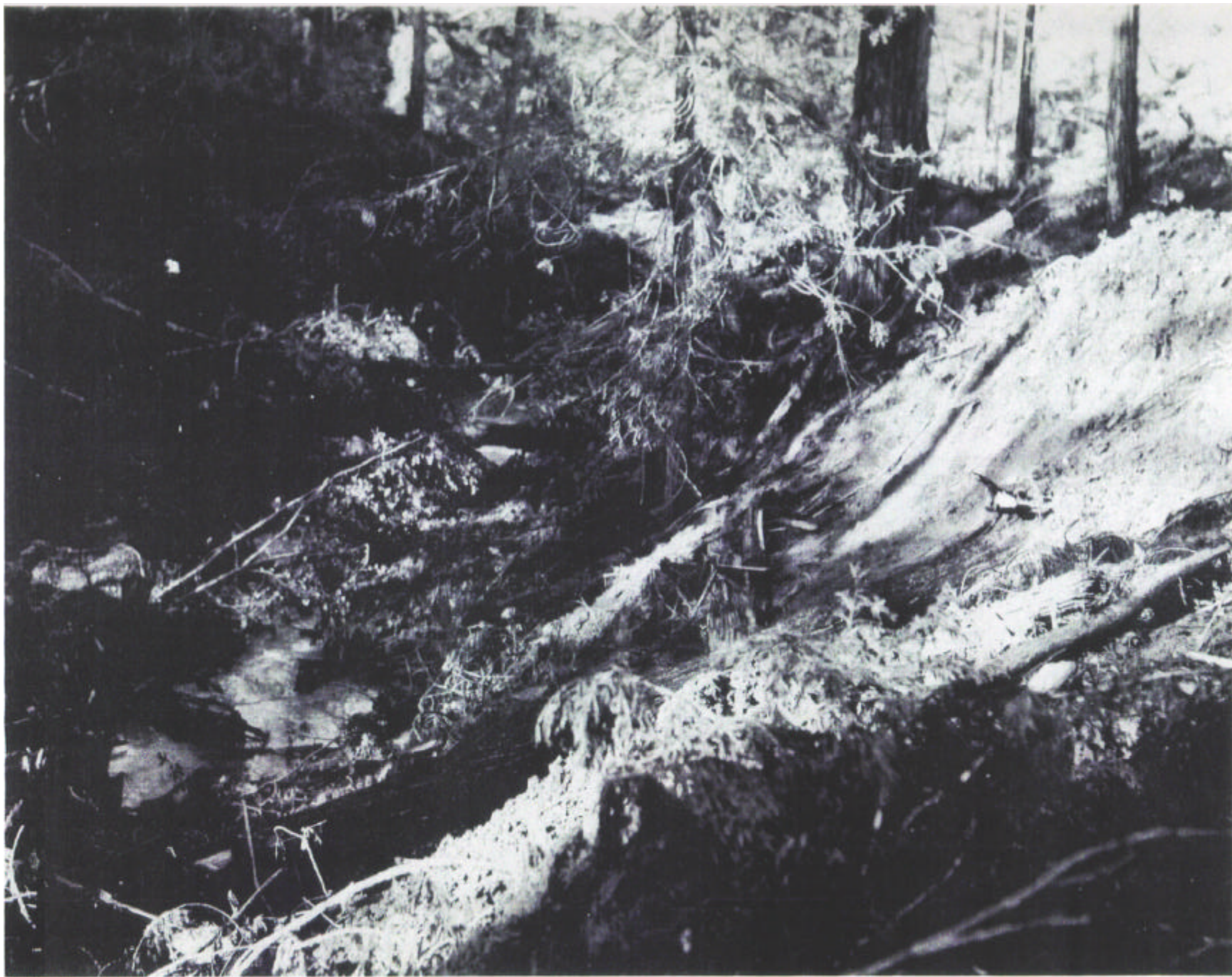
NORTH FORK, GARCIA RIVER, MENDOCINO COUNTY, Nov. 22, 1955. Stream bed and skid road visible at lower left. Road shoulder at right is contributing heavy silt second day after rain. ( Fish and Game photo. )
