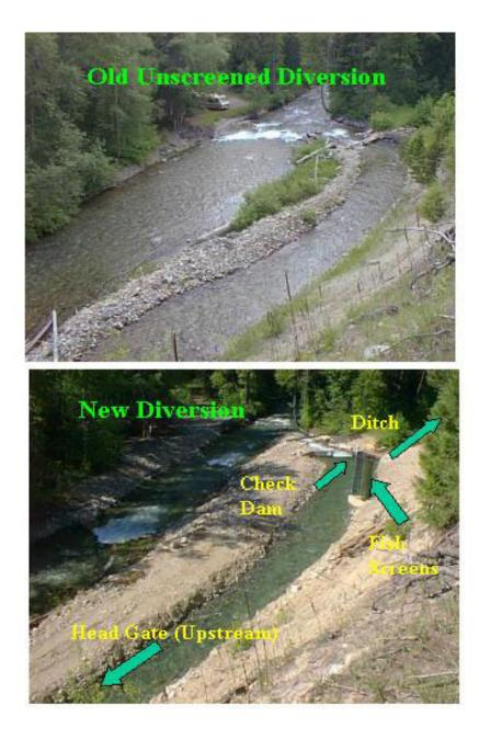
Figure 25. The upper photograph of the Glen Lake Irrigation District (GLID) the unscreened ditch. The lower photograph shows the new diversion side channel, fish screens, and check dam.
