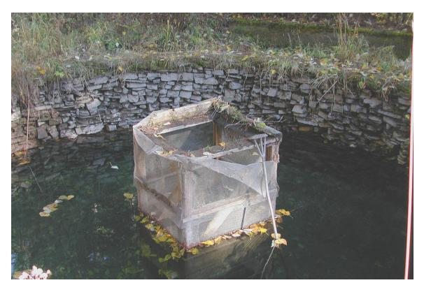
Figure 48. City of Troy water cistern O'Brien Creek, with old outlet pipe screen cover.
