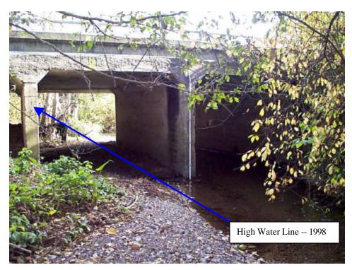
The Redwood Creek Gage was installed in November 1997 on the Highway 1 bridge near Pacific Way. This is a large box culvert, with flow mainly concentrated in two chambers. The stilling well is on the upstream wall directly in the center at high flows. There does need to be maintenance of the site in the winter, as it is possible for debris to get stuck on
