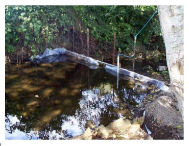
In regards to the Pine Gulch Creek Watershed Enhancement Project, the station will be used for monitoring and enforcement purposes on the low flows. Therefore, we need to install a weir annually or decide to build a more permanent structure that we could use for monitoring low flows. This is actually a realistic alternative, as it is private land, we will be involving the agencies in the process, and it would make sense to have a more permanent monitoring procedure at this site.
