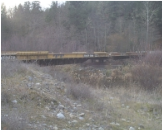
Salt Flat Bridge
