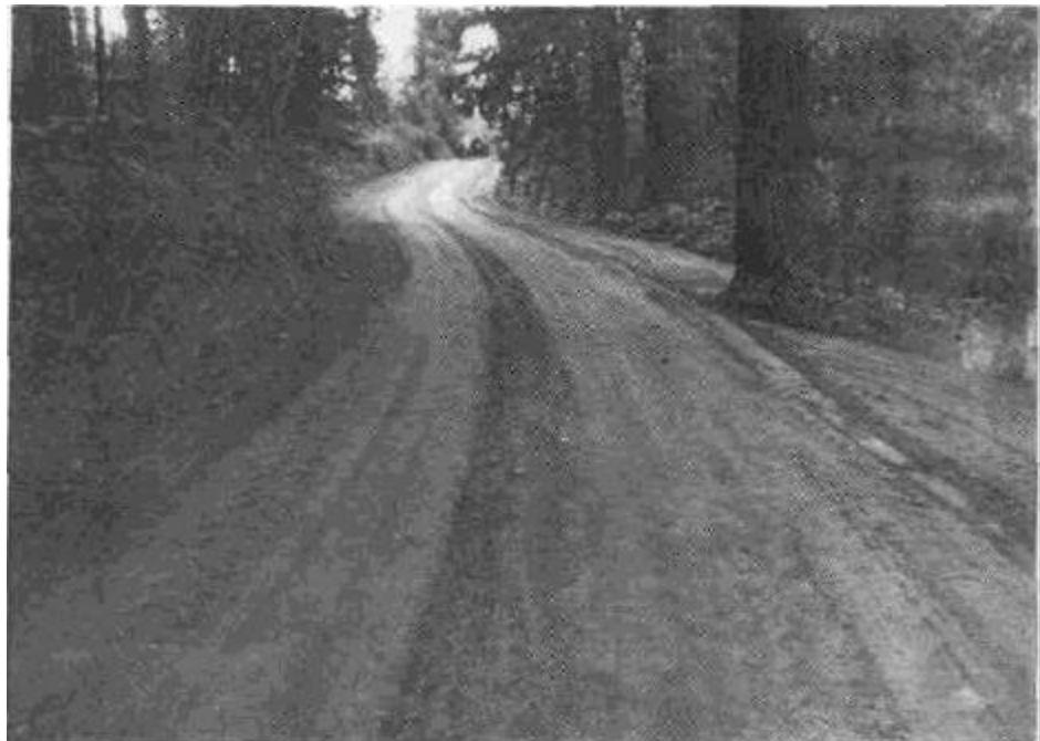
Figure 79. A former insloped road that was regraded and reconstructed to an outsloped configuration. Outsloping was performed to reduce erosion of the ditch and at the outlet of ditch relief culverts, and to lessen maintenance costs. The road bed was lowered about 8 inches along the outside edge of the fill and spoil was graded to cover the inboard ditch. The road was rock surfaced shortly after the photo as taken.
