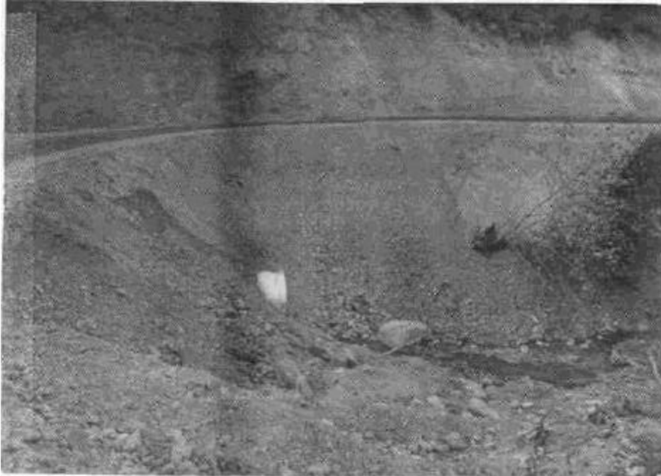
Figure 63. Uncontrolled sidecasting on the approach to this stream crossing has delivered sediment directly to the stream channel. This type of road building is in violation of water quality standards and forest practice regulations.
