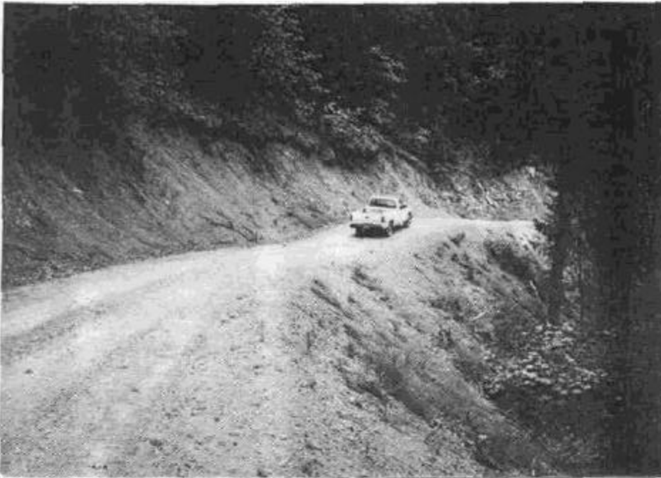
Figure 27a. Rolling dip constructed on a rock surfaced forest road (a). The rolling dip represents a change-in-grade along the road alignment and acts to discharge water that has collected on or is flowing down the road surface.
