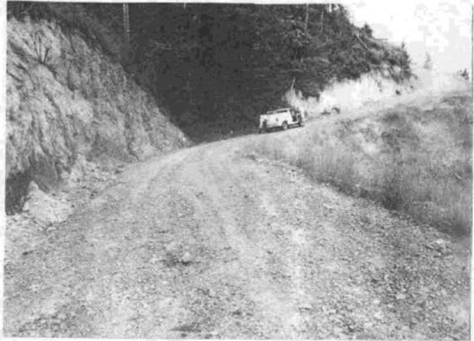
Figure 36. Steeply climbing road crosses a stream channel without changing grade, creating a crossing with a high diversion potential.
