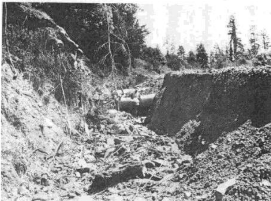
Figure 3. When a stream crossing culvert plugs, or its capacity is exceeded, flood/low can either build up and/low over the road, washing out the stream crossing/ill, or it can be diverted down the adjacent road or roadside ditch, creating a gully on the road and adjacent hillslope. Diverted flow from this plugged culvert has created a large gully in the down-road ditch. Note scale located at plugged culvert inlet. Road prism is to the right.
