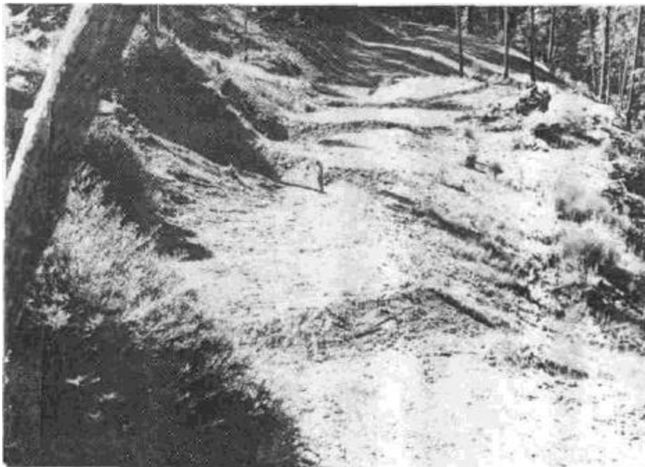
Figure 94. Insloped and ditched roads, especially those with springs and seeps on the cutbanks, should have cross road drains constructed to provide drainage across the alignment. Drains can be installed at wet areas along the cutbank, or at intervals frequent enough to prevent gullying of the roadbed between drains.
