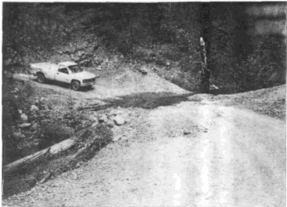
Figure 46. Wet ford on Class II perennial stream. Clean rock aggregate has been imported for the travelling surface and coarse rock armor protects the outer edge of the road bed. It is important that rock aggregate used in a ford be large enough to resist transport during winter flows. Fords should not be used if high winter flows would cut off access to inspect and maintain drainage structures further out the road.
