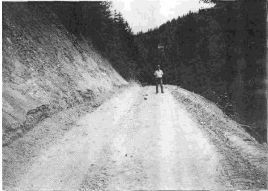
Figure 30. Short road reach where a soil berm has been constructed along the outside edge of the road prism, to prevent surface runoff from flowing over the highly erodible fill. To prevent the road surface from accumulating too much runoff and eroding, the berm can be intermittently breached and a wooden or sheet metal berm-drain used to carry runoff downslope past the base of the erodible fillslope.
