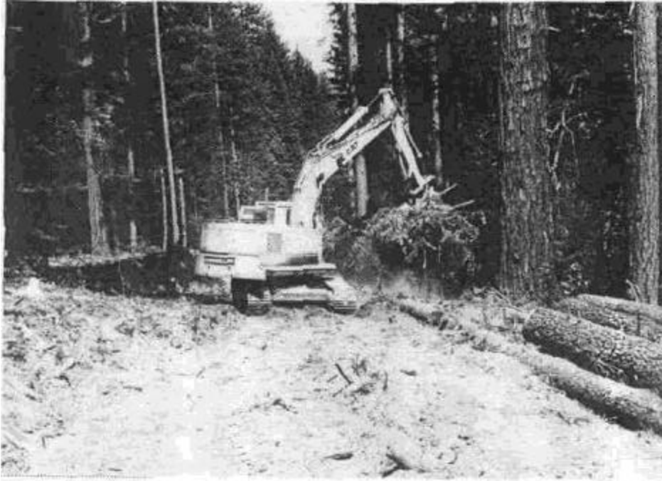
Figure 48. Hydraulic excavators are rapidly becoming the preferred equipment for wildland road construction. Here one is grubbing and clearing the alignment for a new forest road.
