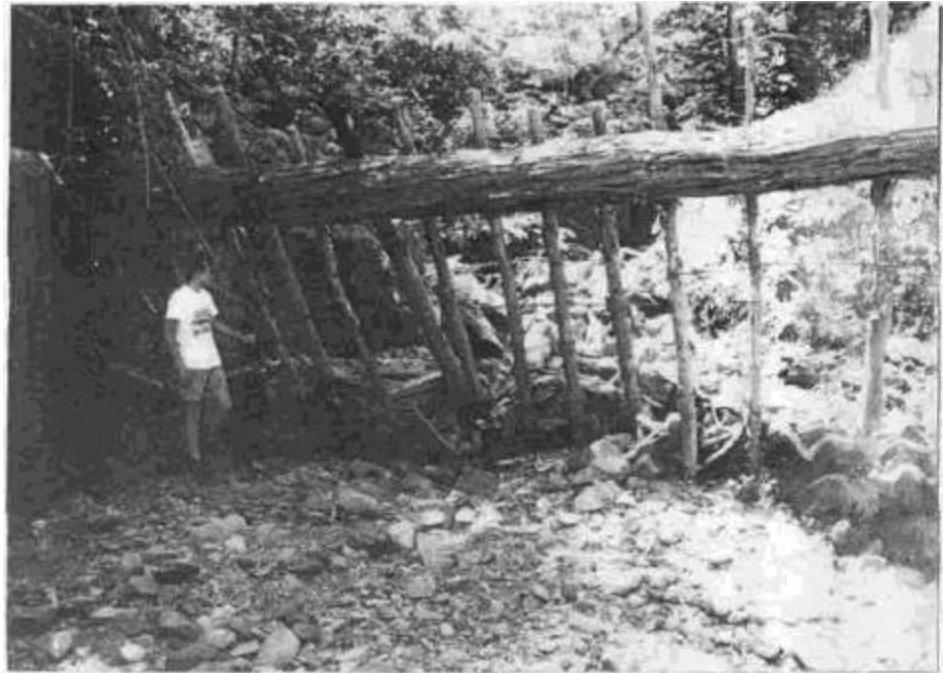
Figure 4 Ib. Limbs and branches floating down the channel are caught before they can plug the culvert inlet.
