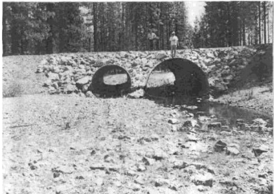
Figure 71. Pipe arch culvert installed in a Class I fish bearing watercourse. Fill face has been rock armored to prevent erosion during high flows. Because of the shallow fill, a second pipe arch culvert was installed to upgrade the crossing to pass the 50-year flood flow.
