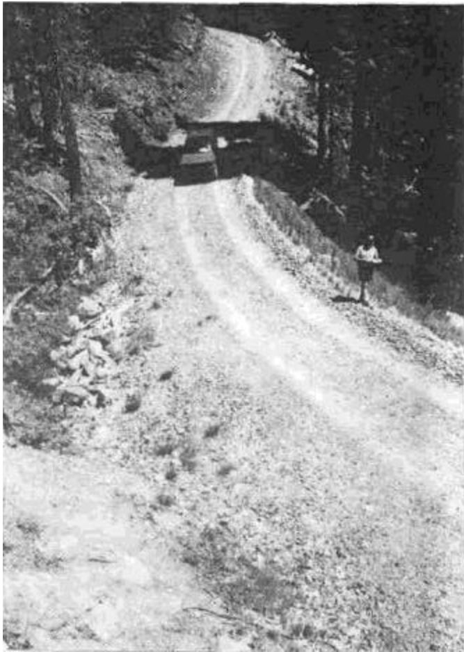
Figure 31. Rock surfaced, insloped road with an inboard ditch. A ditch relief culvert carries ditch/low beneath the road at location "A."
