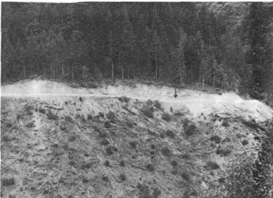
Figure 27b. A side view (b) shows that the rolling dip does not have to be deep to reverse road grade and drain the road surface.
