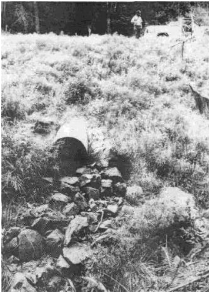
Figure 41d. Culverts and flumes carry high velocity stream flow and outlet areas often need to be protected against erosion by the use of rock riprap .
