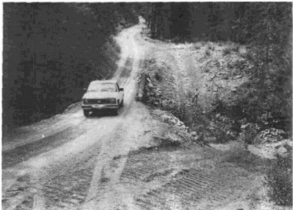
Figure 64. Many bridges built on small forest and ranch roads cannot support or would be damaged by heavy tracked equipment passing over them. For this reason, an adjacent equipment ford is sometimes constructed. These steep fords can erode and deliver sediment to the stream channel if they are not waterbarred, mulched and seeded prior to winter rains.
