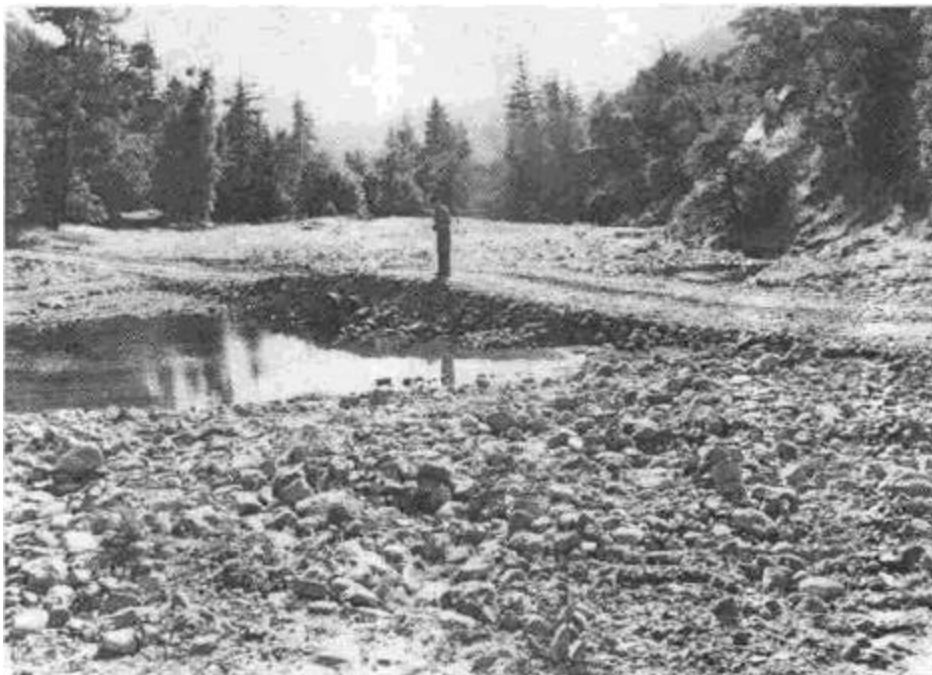
Figure 47. Summer low-water crossing of a Class I perennial stream. Coarse, clean streambed material has been used to ramp up over the flowing water. Two culverts have been installed at water level to allow for uninterrupted flow and the migration of young fish. A temporary bridge crossing should be used where migrating adult fish need to pass beneath the crossing. Low water crossings should be removed before the first fall rains.
