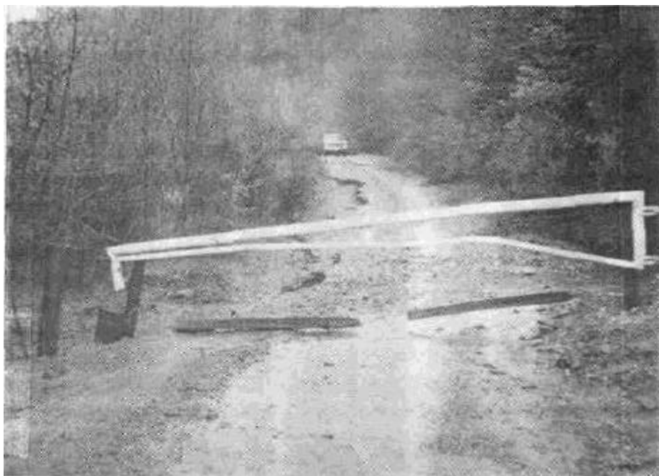
Figure 90. Gating a road closes it to unauthorized traffic, but does nothing to protect the road from erosion. Scarps in the road fill behind this gate signal a slope failure that threatens to deliver sediment to an adjacent fish-bearing stream.
