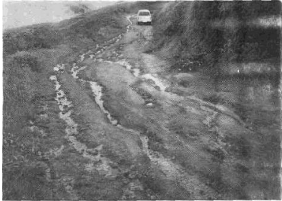
Figure 81. Surface runoff problems cause by winter use of a bermed, unsurfaced road. Running surface is rutted and this acts to collect runoff and cause additional erosion. Lack of waterbars or rolling dips, together with the graded berm along the outside edge of the road, now acts to keep surface runoff on the road bed. Annual grading can produce an outside berm of soil and rock that should be pulled (graded) back onto the road surface before winter rains.
