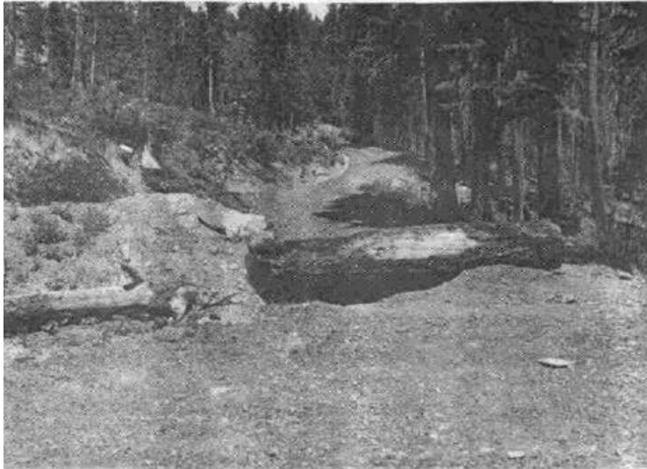
Figure 86. There are a variety of ways to close a road to off-season traffic, but it should always be remembered that barricading the road does not by itself prevent erosion along the alignment. Gating closes the road to unauthorized traffic but still allows for winter maintenance and inspections. If barricades or physical barriers are used, they must be removed with heavy equipment before maintenance activities can be performed. They should not be used on roads which have stream crossings since these need to be inspected and maintained during storms.
