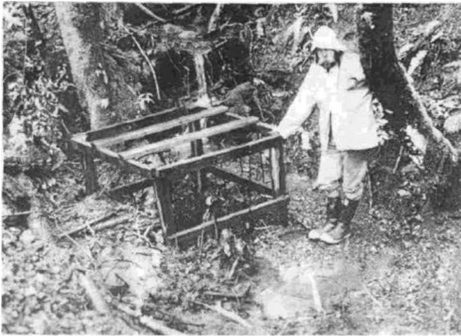
Figure 88. Most culvert maintenance involves cleaning the inlet of sediment or woody debris. This trash rack, built over the culvert inlet, was nearly plugged during a normal winter storm. Without storm maintenance inspections such minor culvert plugging often ends up causing severe gully erosion when the stream/low is diverted out of its channel, or it flows over and erodes the stream crossing/ill.
