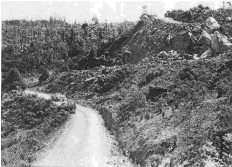
Figure 77 a. Access road and rock pit before (A) and after (B) reclamation. Exposed areas have been reshaped and covered with soil to promote revegetation. The area was then mulched, seeded and planted. Reclamation work was performed using an excavator and large bulldozer.
