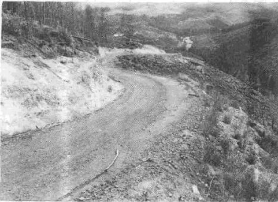
Figure 54. Rock surfaced, outsloped forest road constructed by hydraulic excavator. Note the absence of an outside road bench which would otherwise collect and concentrate surface runoff on the road prism.
