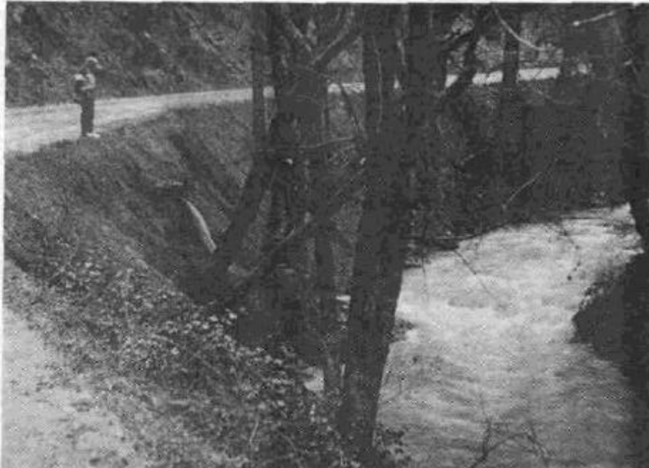
Figure 10. Because of our increased awareness of the potential impacts to streams in a watershed, some roads which were built in the past would probably not be built in the same locations today. In this example, a side-cast-constructed road was built alongside a large, fish-bearing stream and ditch relief culverts still discharge muddy road runoff into the channel during storms.
