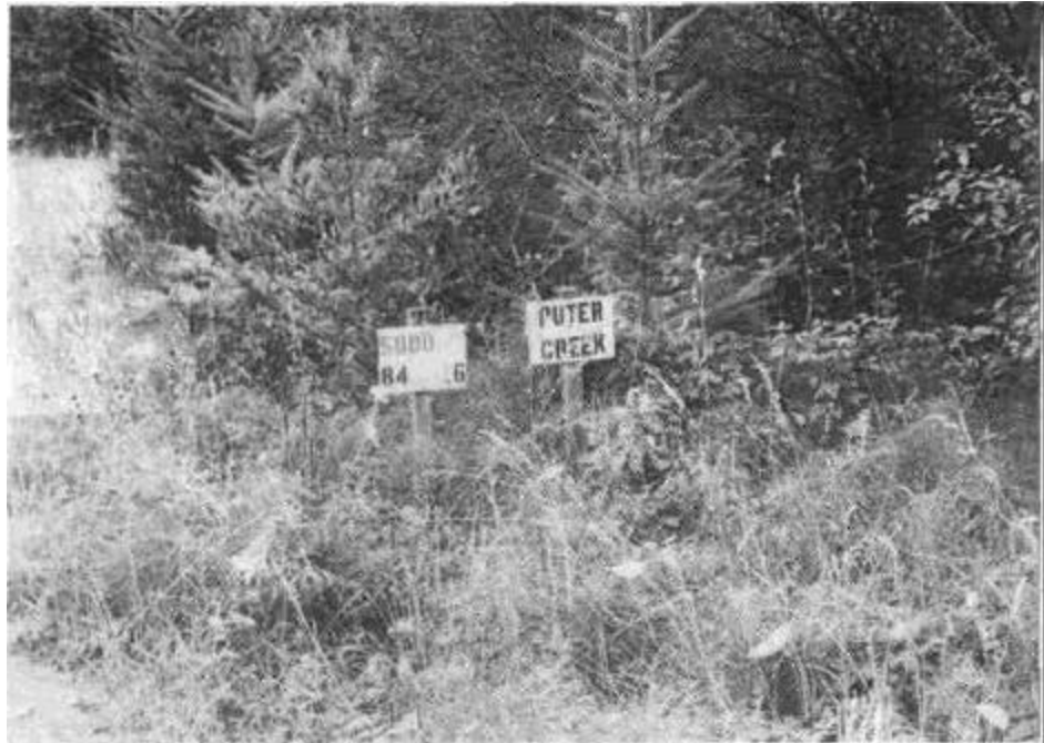
Figure 84. Culvert signing is an integral part of developing a culvert and drainage structure maintenance plan. Included at this crossing are the stream name (Puter Creek), the name of the road (5000 Road), the diameter of the culvert (84") and its location (0.6 miles from the beginning of the road). The signing can also be color coded (e.g., green, yellow, red) to indicate whether or not it is prone to plugging or other maintenance needs.
