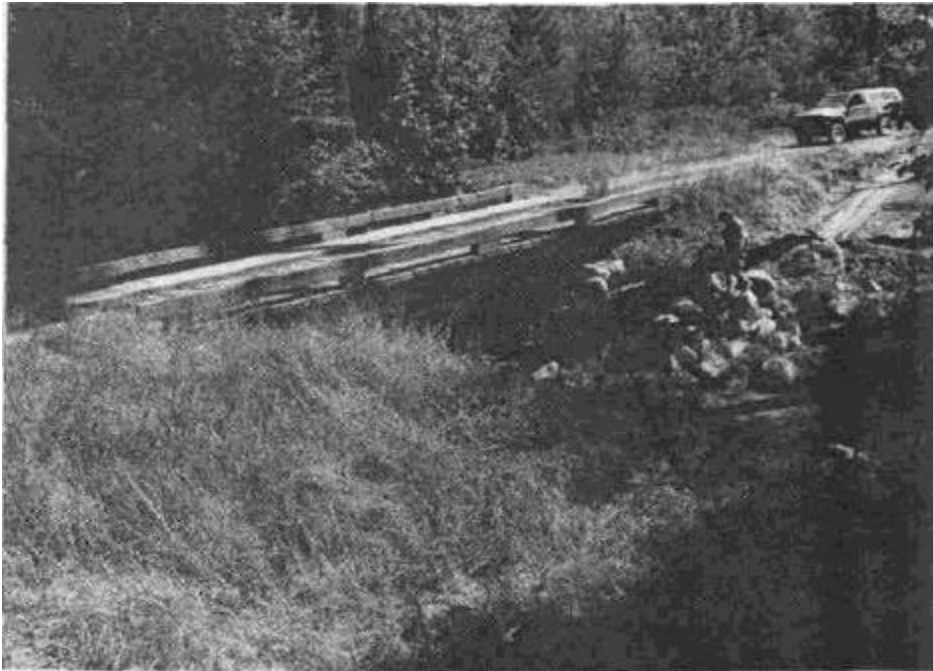
Figure 43b. If possible, it is usually best to span the channel without using center supports and to build abutments well out of the flood zone of the channel. Abutment areas exposed to flood waters should be armored to protect them against erosion. In practice, abutments should be built up and out of the flood zone so they do not restrict channel flood capacity.
