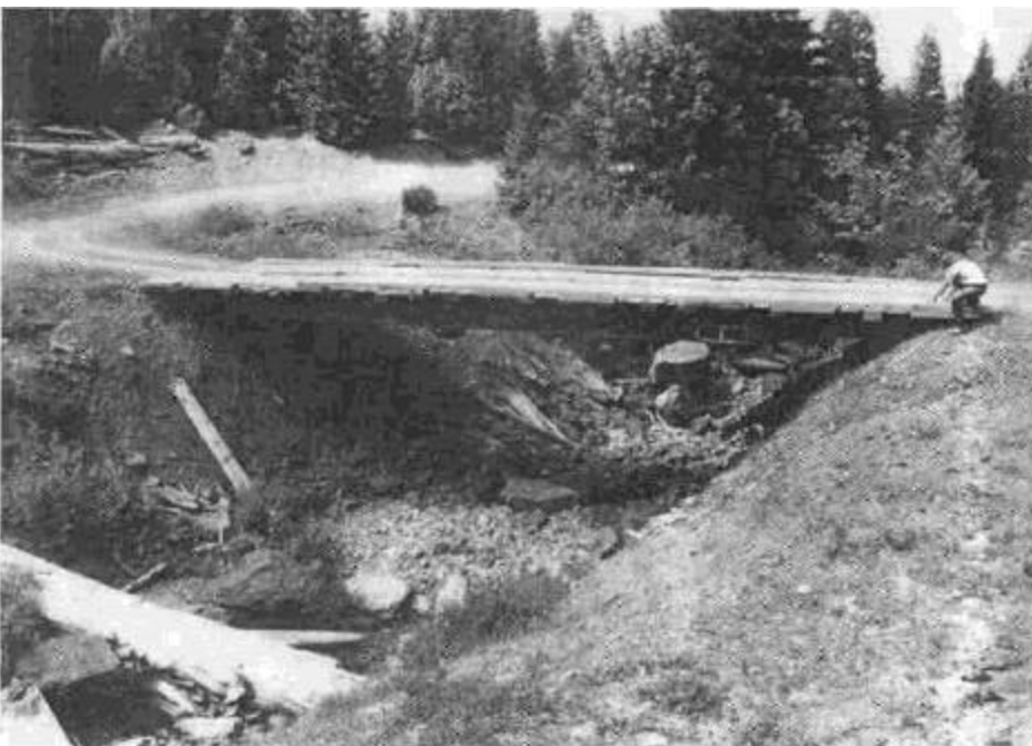
Figure 66. Railroad flatcar bridge correctly crosses stream channel at a 90° angle, but bare, unprotected soil abutments are subject to erosion during high flows. Low, summer stream/low goes subsurface under the bridge because of extra sediment in the channel bottom at the crossing site.
