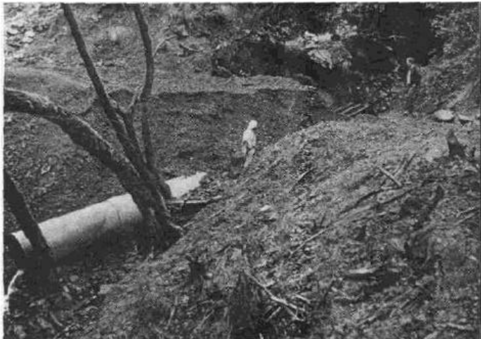
Figure 2. This stream crossing "washed out" (eroded) when the culvert plugged and streamflow scoured through the road road fill. Sediment was delivered directly to the stream system as the fill eroded. Stream crossings and culverts need to be properly designed and maintained to minimize the potential for such failures.
