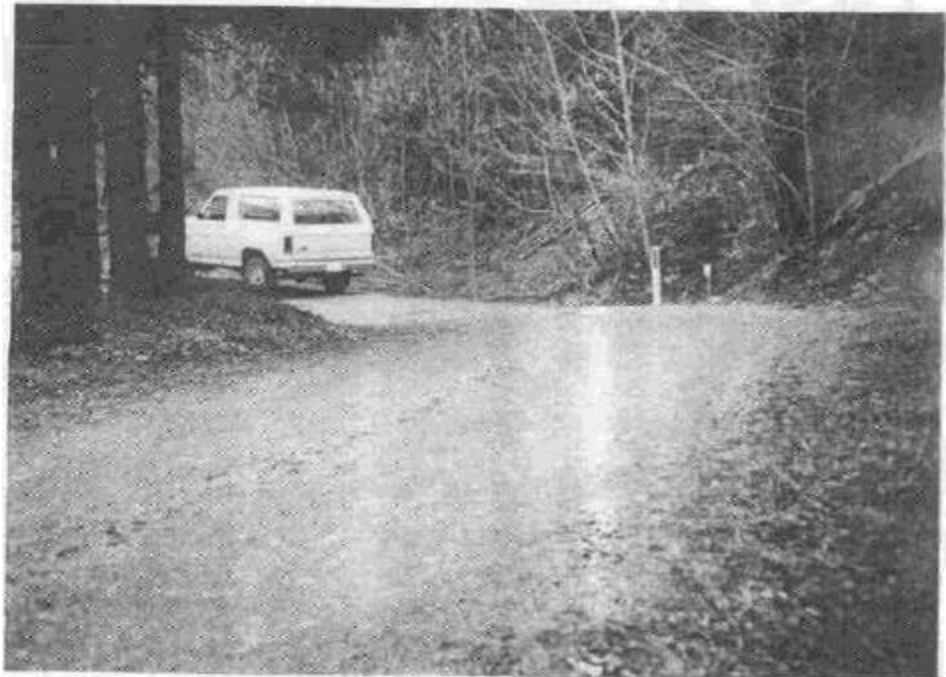
Figure 37. A gradually climbing road changes grade over the stream crossing, thereby eliminating the possibility for future stream diversions.
