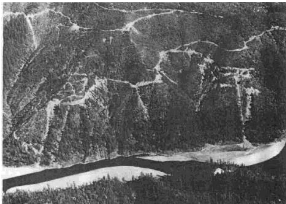
Figure 4. Sidecast road construction on steep or unstable stream-side slopes and canyons has a high potential/or causing landslides which deliver sediment to downslope stream channels.
