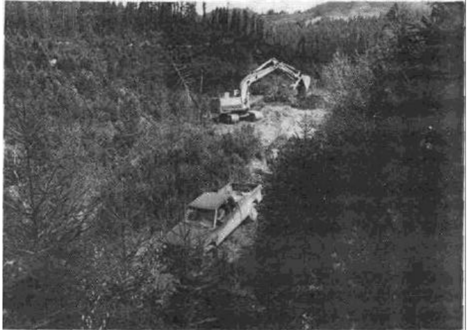
Figure 93a. Excavation of unstable landing fill on a road scheduled for permanent closure: (a) before excavation.
