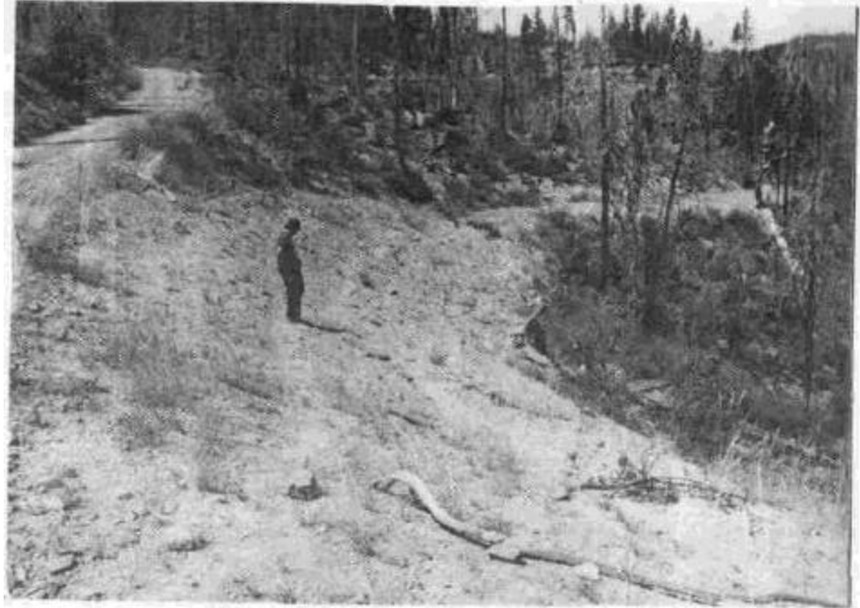
Figure 87b. Outsloping should only be used on temporary roads where all stream crossings have first been removed.
