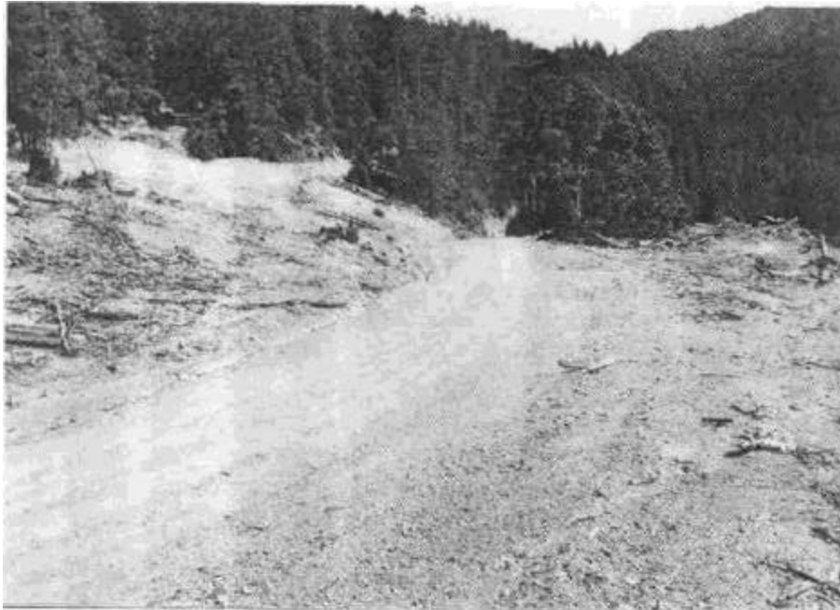
Figure 60. Typical spoil disposal site (uphill side of road) for endhauled spoil materials from a full bench road construction site. Spoil disposal site is located on a broad, gently sloping, dry ridge. Material is dumped, spread, compacted (by bulldozer) and seeded, mulched and planted.
