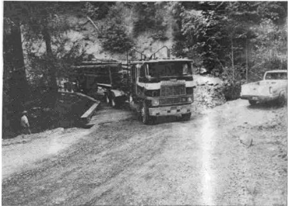
Figure 44. This railroad flatcar bridge has been structurally modified to allow for some truck turning on the bridge deck. Deeply incised stream channels with steep sideslopes would require extensive hillslope excavation if a straight approach was utilized. The underside of this bridge can be seen in Figure 65.
