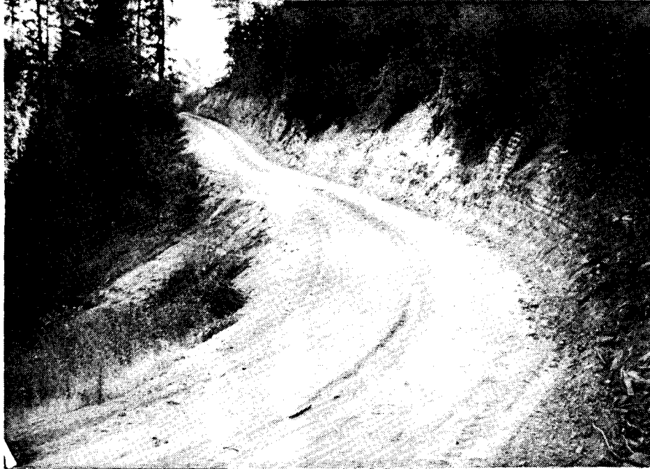
Figure 16. Full bench road. The height of the cutbank, the slope of the natural hillslope and the small amount of sidecast indicates that this road is full bench and cut entirely into native hillslope materials. Note that the road is outsloped with rolling dips and no inboard ditch.
