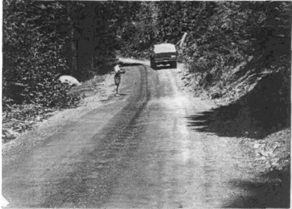
Figure 26. Well built outsloped road displaying minimum cut, smooth free draining surface, no outside berm and rolling dips to help disperse surface runoff.
