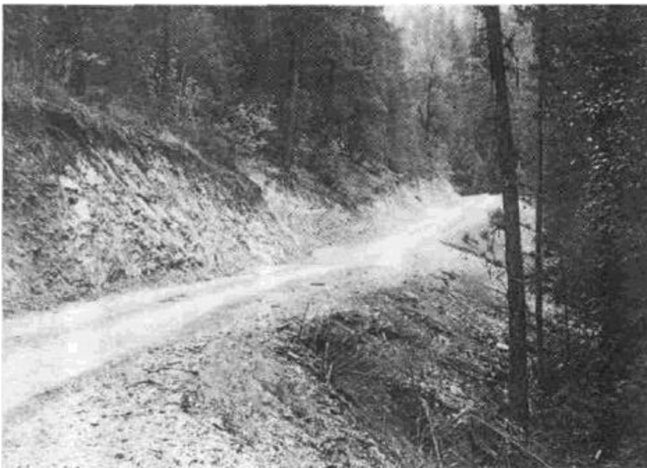
Figure 74. Several rolling dips in close succession on a rocky, outsloped road built across moderately steep terrain. As road grade increases, rolling dips need to be spaced more closely.
