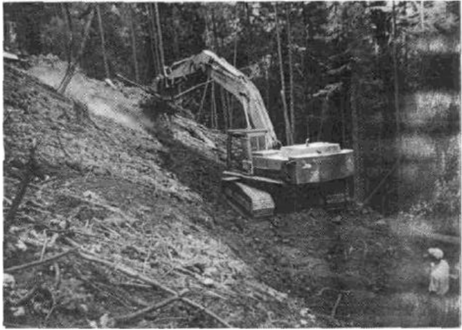
Figure 51. Each step of the way, the excavator clears vegetation and grubs the slope surface in front of it before it excavates and extends the road bench. Excavated soil from the new segment of road bench is placed and compacted on the grubbed slope below the new segment of road bench. Cleared vegetation placed along the base of the future fillslope helps contain erosion from the exposed fill.
