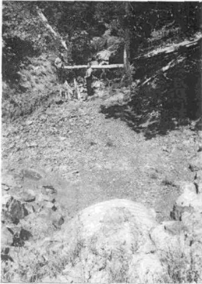
Figure 41a. Trash racks at culvert inlets and energy dissipation at culvert outlets are methods of preventing erosion of the stream crossing fill. The most effective trash rack is one placed across the channel just upstream from the culvert inlet.
