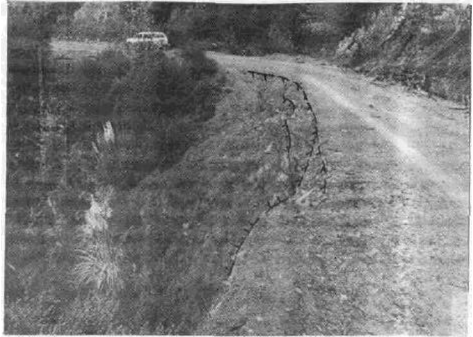
Figure 89a. Unstable fill along the outside edge of active roads can often be excavated and removed without impeding normal traffic. In photo "a," 12 inch scarps bound unstable fill that threatens to fail on steep slopes above a perennial stream.
