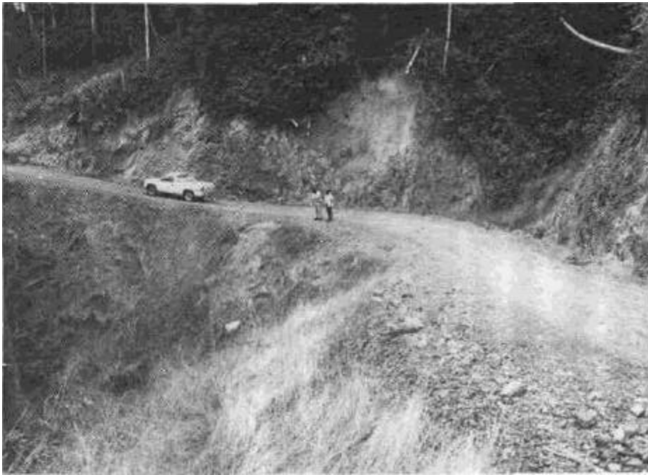
Figure 78. Mulching and seeding are effective methods for controlling surface erosion from bare fill slopes. Mulch protects the soil until the grass and vegetation is firmly established. However, because it decomposes rapidly, straw mulch is effective for only the first year. After that, well established vegetation should provide the needed protection.
