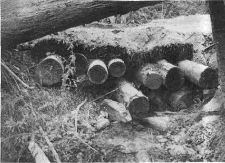
Figure 73. End view of a temporary stream crossing. First, a culvert was placed in the channel bottom. Then cabled logs were placed on top, followed by a thick layer of straw and then soil material for the temporary running surface. The materials comprising the temporary crossing are easily removed upon the completion of operations.
