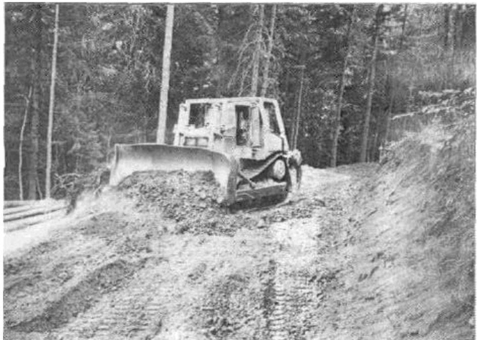
Figure 52. Behind the excavator, a bulldozer is used to prepare the final subgrade, surface shape and width of the new road.
