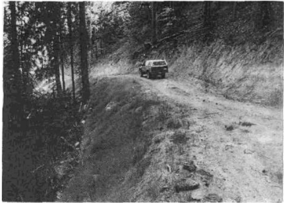
Figure 76. Newly constructed, outsloped forest road with accumulated line of slash, called a filter windrow, at the base of the fill to catch soil eroded from the fill slope. Slash should be placed at the base of the fill, and not Incorporated into the soil material. This fill has been straw mulched and is covered with a thick stand of grass. Filter windrows are most important to install where roads approach and cross stream channels. Note how the road conforms to the topography of the land and incorporates rolling dips at natural swales to shed surface runoff.
