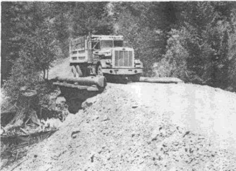
Figure 68. Wheel guards on a railroad flatcar bridge signal the driver that he is too close to the edge of the bridge. Note how the approaching road slopes up to the bridge so that road runoff does not flow onto the bridge deck.
