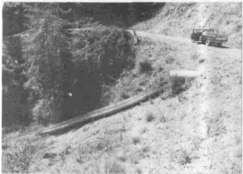
Figure 41 c. Culvert trash racks which are constructed right over or against the culvert inlet should be avoided because they can plug and, in turn, prevent streamflow from entering the culvert inlet. Culverts that are not set into the bed of the original channel and would discharge runoff onto the road fill need to be extended with an elbow and full round culvert extension, or with a flume (in this case a half-round culvert) past the base of the erodible fill.
