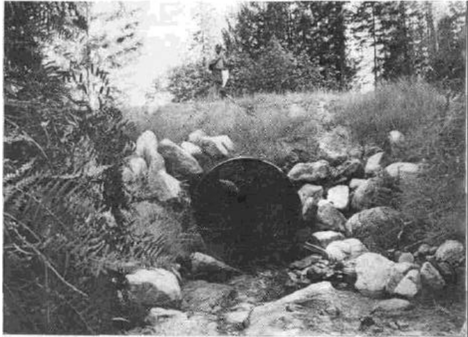
Figure 70. Culvert installation on a low gradient Class II (non-fish bearing) watercourse. Culvert is set slightly into the original streambed and inlet is armored to prevent erosion. Roadbed dips into and out of the stream crossing and trash rack (not visible) has been installed just upstream from the culvert inlet.
