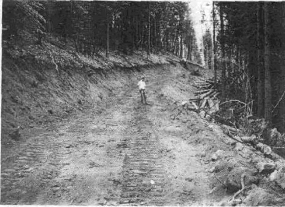
Figure 53. New road constructed by excavator and bulldozer. Logs harvested from the right-of-way have been placed on top of the filter windrows and will be hauled away later.
