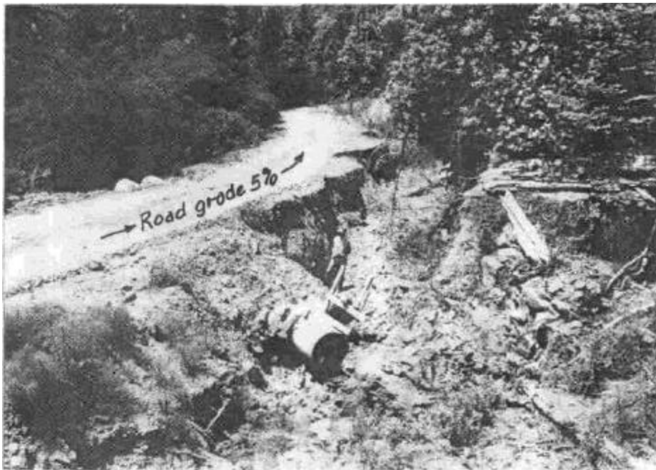
Figure 35. Double culvert stream crossing showing the result of a stream diversion that occurred during a winter storm. The road slopes to the distance at about 5 percent, so when the culverts plugged with debris, water flowed down the inboard ditch and created the large diversion gully.
