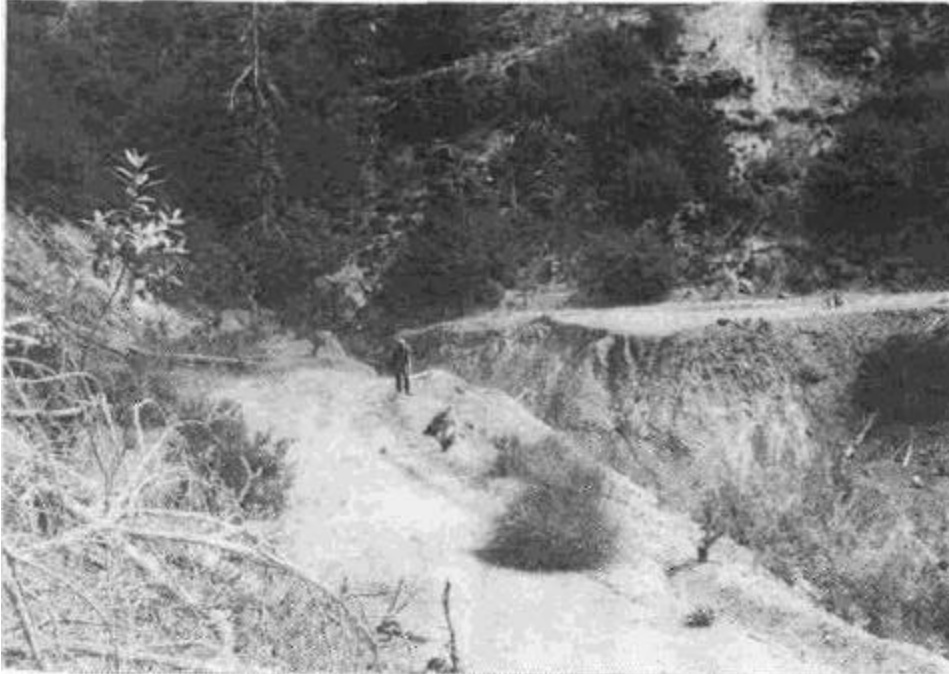
Figure 80. Under-designed or unmaintained stream crossings on older roads are prone to failure during large storms. During road reconstruction, stream crossings should be redesigned for the 50-year flood flow. Under-designed culverts and Humboldt log crossings should be removed and upgraded.
