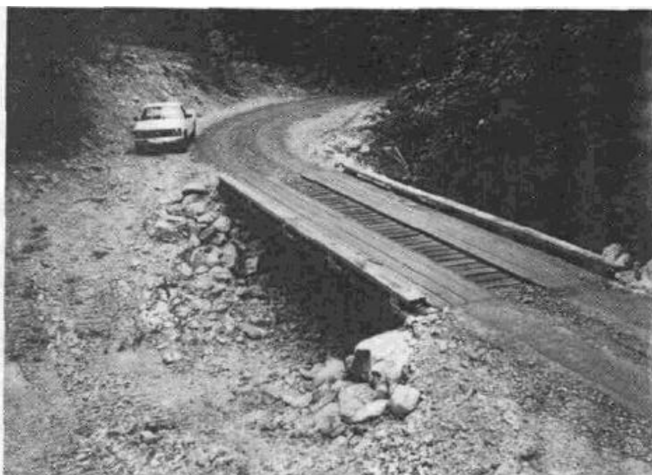
Figure 42. Low cost railroad flatcar bridges can be used for temporary crossings of incised stream channels, or they can serve as permanent watercourse crossings.
