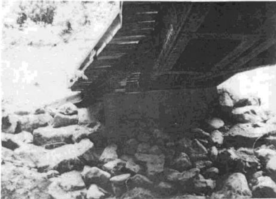
Figure 65. Bridge abutments can be built of logs, piers, concrete pads and other supports. This abutment is a precast concrete support that was fabricated off-site and installed when road construction reached the crossing location. It is tied into the adjacent slope with cables secured to buried "deadmen."
