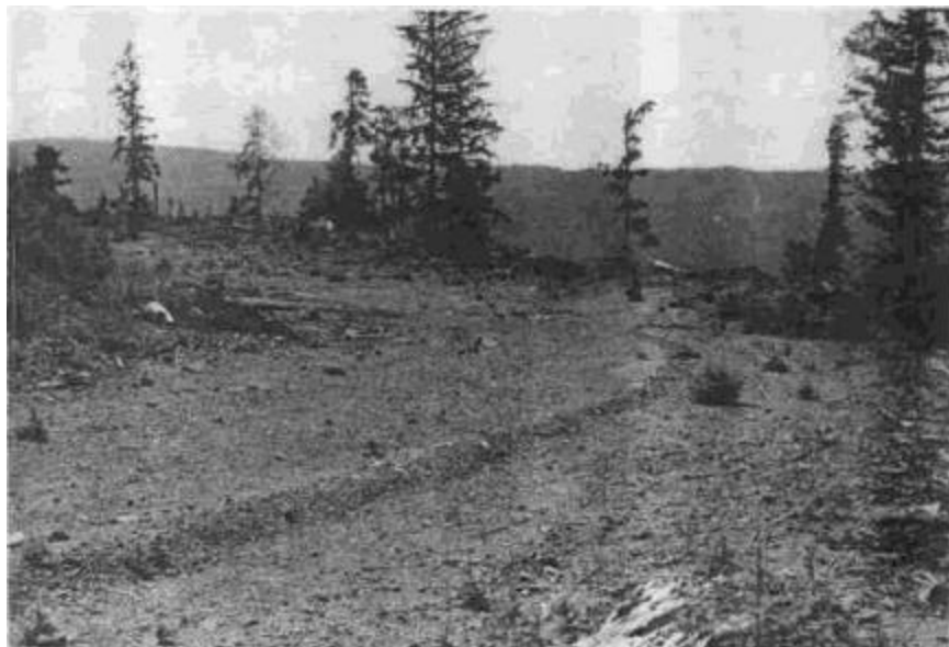
Figure 95a. On forest roads which are to be formally closed, rather than just "abandoned," the roadbed can be returned to forest production by ripping and disaggregating the surface and then planting with trees. Photos "a" and "b" show a road/landing before and after decompaction. This simple, inexpensive process also helps reduce runoff from compacted areas.
