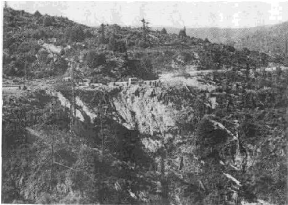
Figure 82. Excess sidecasting on forest roads and landings that are scheduled for reconstruction should be excavated before it fails and is delivered to a stream channel. Often, potentially unstable spoil can be recognized by cracks and/or scarps along the margins of the road or landing surface.
