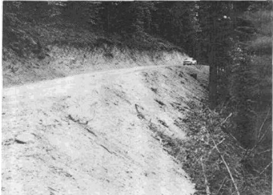
Figure 49. Road constructed by cutting and sidecasting. A row of slash and organic debris along the base of the sidecast slope can help catch and filter soil eroded from the loose slope. Soil should only be sidecast onto gentle or moderate slopes that have been cleared and grubbed of vegetation, and where material cannot be eroded and delivered to a stream .
