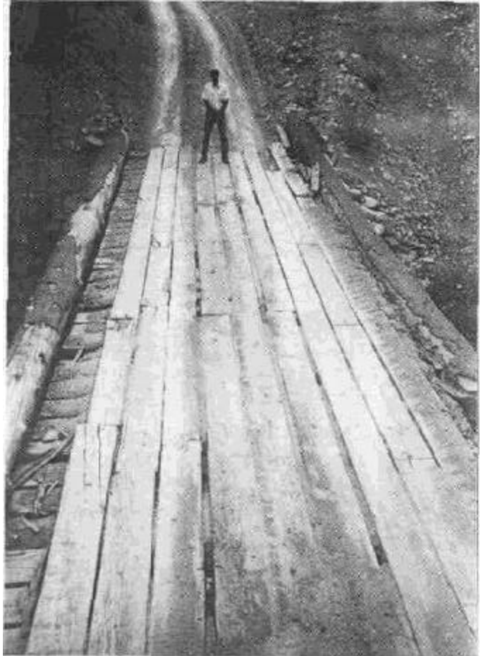
Figure 67a. The segments of road which approach a bridge should not drain onto the bridge surface. Otherwise, soil eroded from the adjacent road surface can be carried onto the bridge and into the stream.
