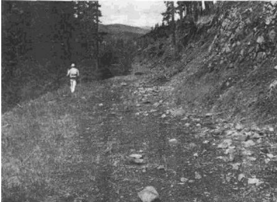
Figure 9. Temporary roads are often spur routes constructed off permanent or seasonal roads that provide short-term access to watershed areas. They are usually outsloped, unsurfaced and used only during dry soil conditions. All stream crossings need to be physically excavated and removed upon the completion of operations or prior to the onset of the winter period (October 15 for forestry roads). In forested areas, the road bed can be planted with trees to return the site to productivity.
