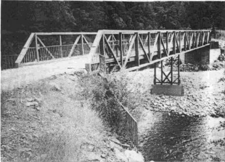
Figure 45. It is important that all bridges used to transport vehicles and equipment be properly designed or evaluated by a structural engineer before they are put into use. This large, reinforced bridge was fabricated from four railroad flatcars with a center pier support that can be folded up under the bridge during winter flood flows.
