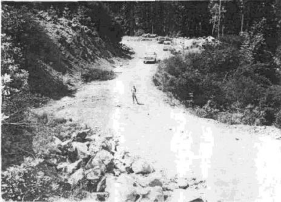
Figure 92a. Stream crossing on a temporary road before (a) and after (b) it was excavated and the road was closed (person is standing over the axis of the stream channel). Since the road bed is still intact everywhere but at the stream crossings, it can be reopened by simply reinstalling the culverts. In the meantime, no road maintenance is required.
