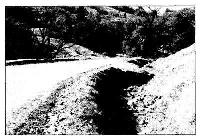
Figure 16. Enlarged Kelly Road ditch where small stream has been captured
